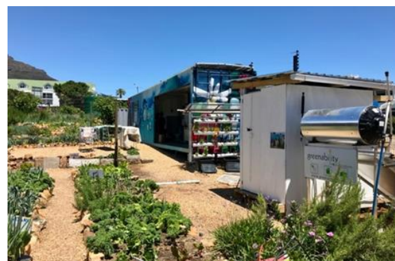
Figure 17: Expansion of the LaundReCycle with a shower and hydroponic system with the aim to explore wider greywater reuse applications
