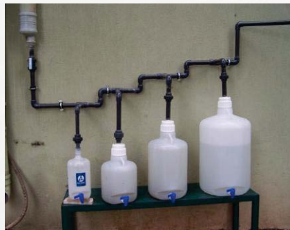
RW sampling system from roof
